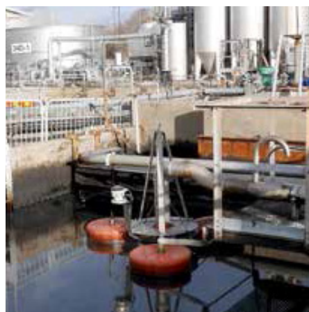
Equipment: Ultra-Surf Cleaner-400 Capacity: 8,000 liters (2,113 gal) per hour Purchased: 2002
