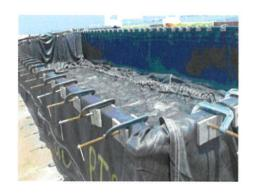
Excess water drains from the Eco - b a g through the small pores in the geotextiles resulting in effective dewatering and efficient volume reduction of the contained material. This volume reduction allows for the repeated filling of the Eco-bag.
